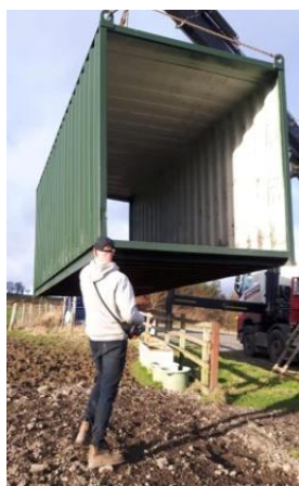
Taking delivery of our great new field shelter.
